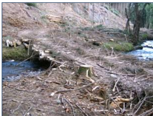
Plate 4-1 and Plate 4-2 Examples of temporary stream crossings
